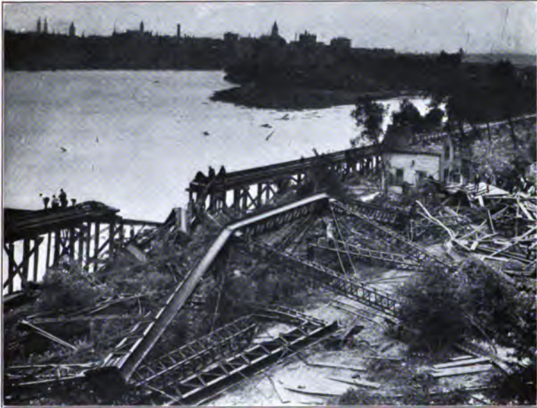
FIG. 1.—SMITH AVE. VIADUCT. VIEW LOOKING SOUTHWEST. SHOWING PART OF SHORE TOWER, AND ALSO RAILROAD TRESTLE CUT THROUGH BY THE FALLING TOWER.
